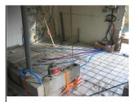
About in the middle of part 1 is the beginning of a wall that has to support the roof. The tiles we are going to put up are a lot heavier than the corrugated steel plates, and since we do not want the roof to collapse or even bend, we had to make this support.
