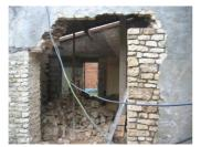
openings are made. The sides are masoned with the outcomming "pierres" as a mould to create a piler on which the lintel will be putt.
